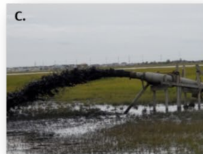
Placement at (A) Gull and (B) Sturgeon Island. (C) Dredged slurry being pumped on southern Gull Island. (D) Innovative sediment distribution pipe being utilized as part of the Sturgeon Island placement.
