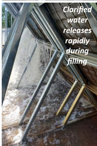
ODNR's Dredging Team hydraulically-pumps slurried sediment filling the GeoPool in the shadows of idle steel mill—consistent solids percentage and flow found to be critical to polymer dose and function
