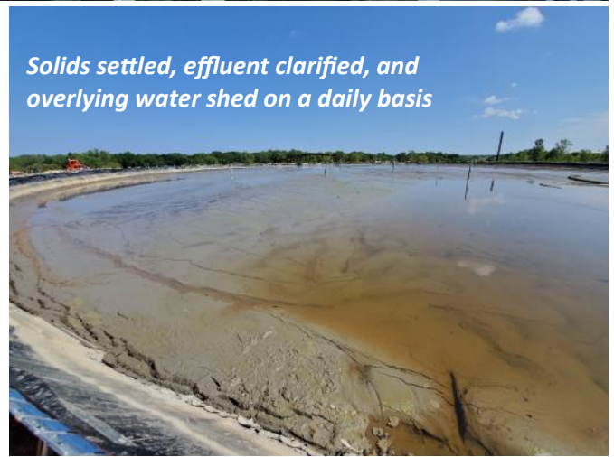
ODNR's Dredging Team hydraulically-pumps slurried sediment filling the GeoPool in the shadows of idle steel mill—consistent solids percentage and flow found to be critical to polymer dose and function
