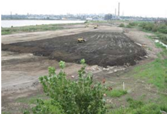
Moisture conditioning of PDM
