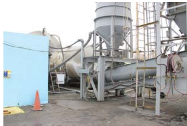
Pneumatic pozzolan metering system
