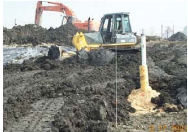
Placing PDM layer at landfill
