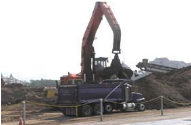
Loading of PDM in truck
