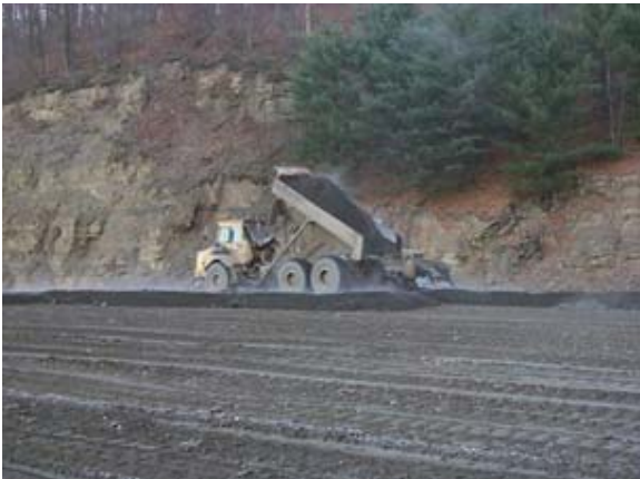
Placing cured PDM in lifts
