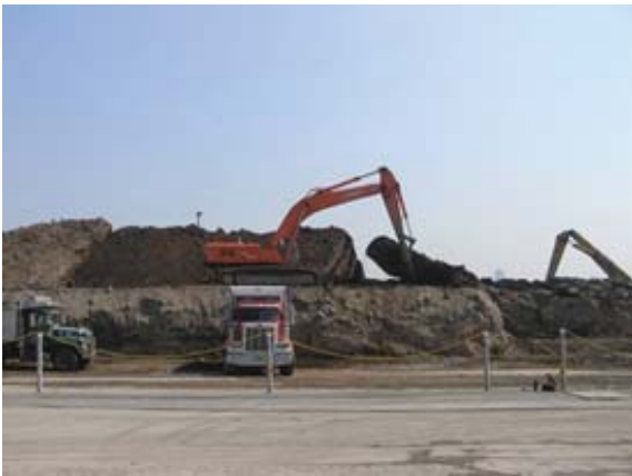
PDM curing operation
