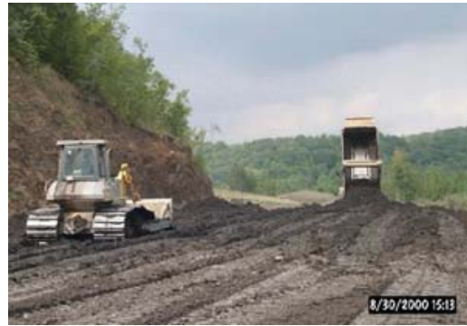
Placing PDM on highwall
