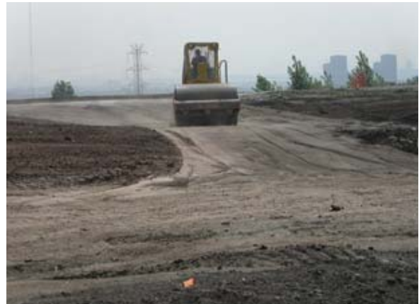
Compaction of PDM grading layer
