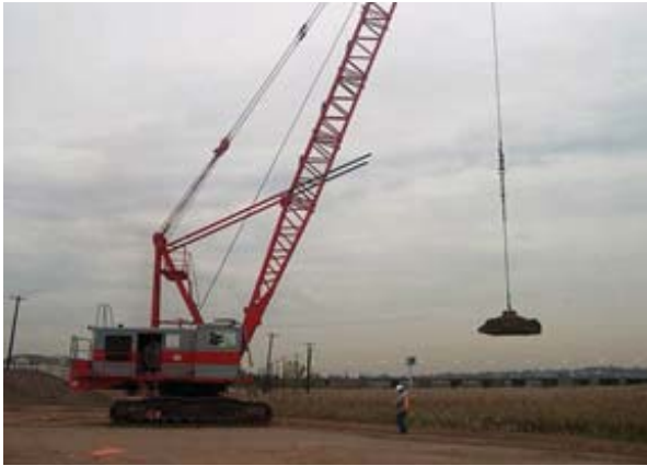
Dynamic compaction of waste
