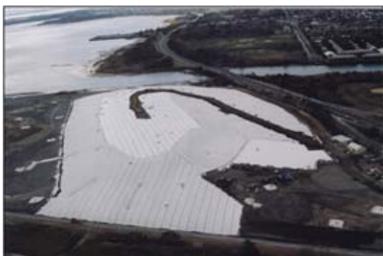
Geotextile membrane on landfill
