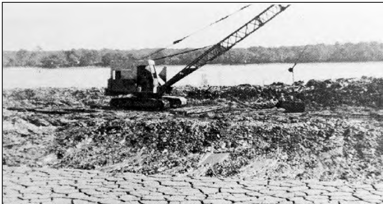
Figure 4-32. A Small Dragline on Mats, Working on a Berm, Deepens a Shallow Perimeter Trench
