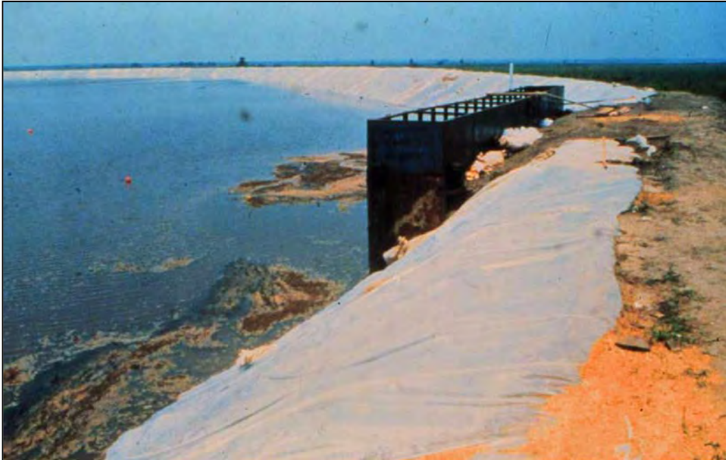
Figure 4-19. Rectangular Weir (1)
