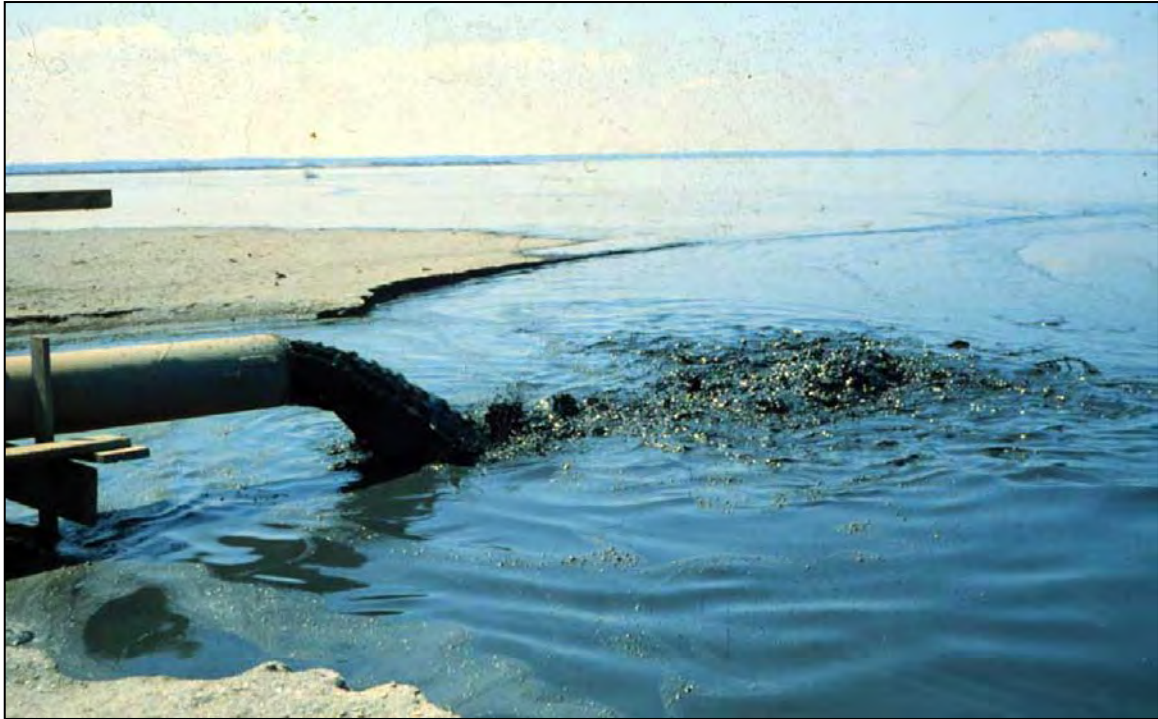
Figure 4-6. Typical CDF Hydraulic Inflow from a Cutterhead Pipeline Dredge
