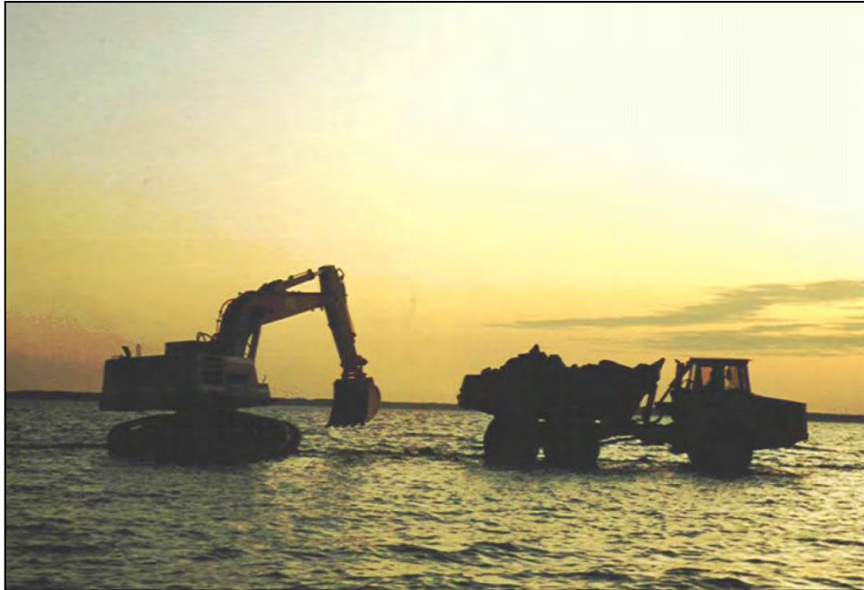
a. Construction of the Riprap and Dredged Material Detached Breakwaters to Break Wind Fetch and Wave Energy, Approximately 125 m (400 ft) Offshore in Shallow Water at Eastern Neck National Wildlife Refuge
