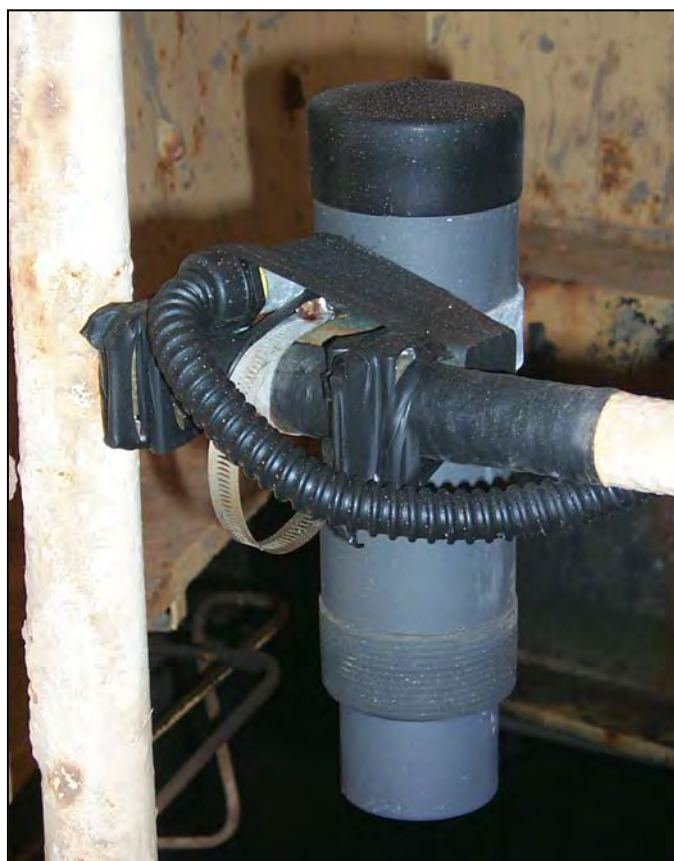
Figure 2-45. Acoustic Hopper Level Sensor
