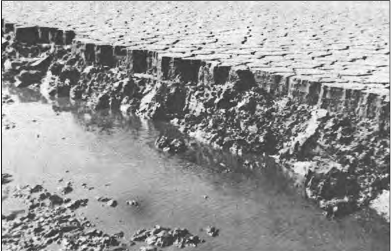
Figure 4-34. Desiccation Crust Adjacent to the Perimeter of a 1-1.5 m (3-5 ft) Deep Drainage Trench
