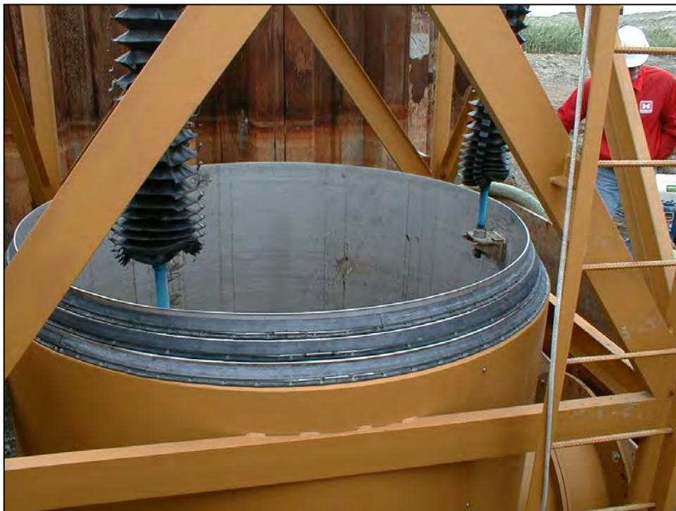
b. Closeup of Adjustable Weir
