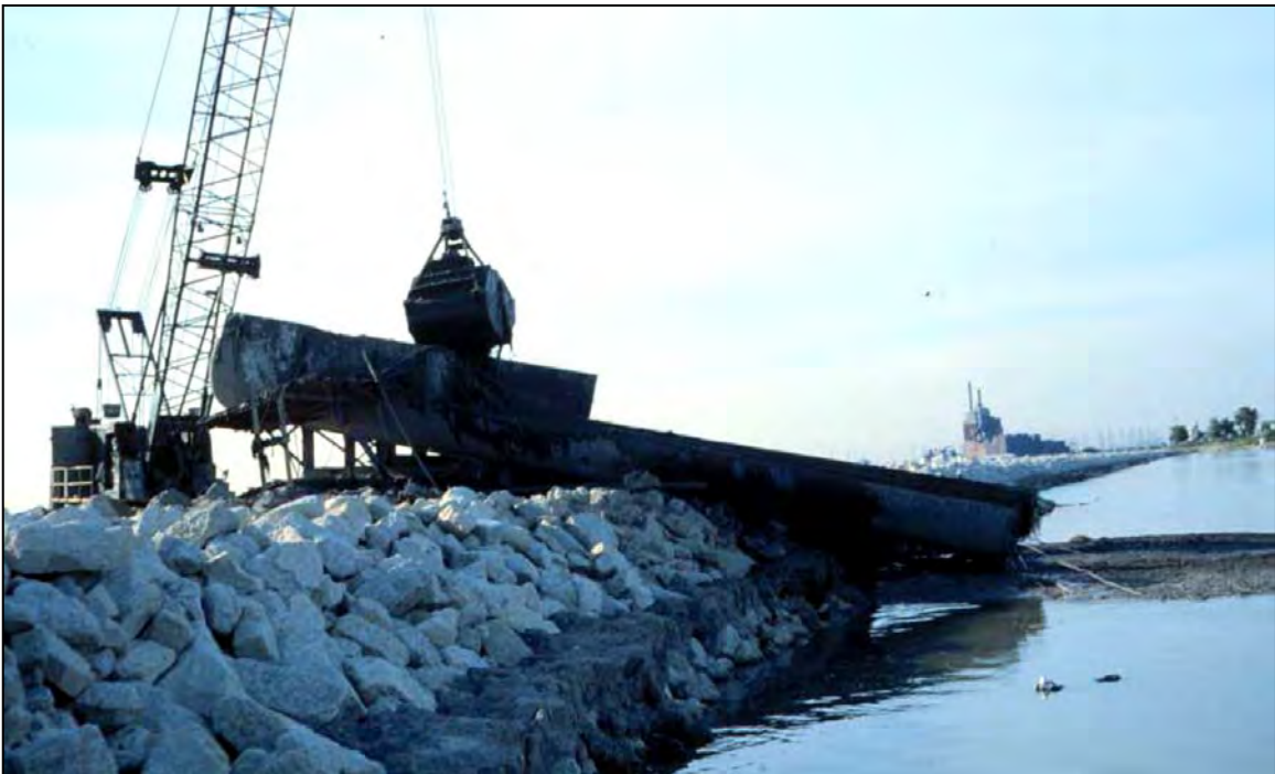
Figure 4-11. Placement Using a Chute Fabricated from Railcar Tanks for Direct Mechanical Placement into a CDF
