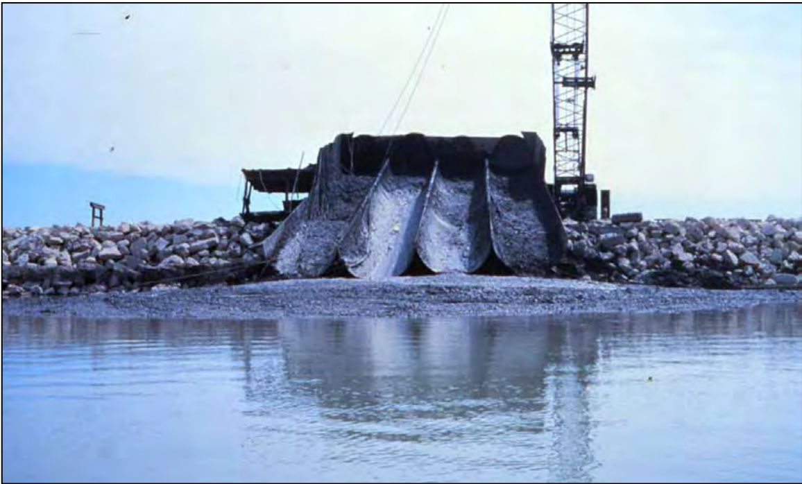
Figure 4-10. Chute Fabricated from Railcar Tanks Used for Direct Mechanical Placement into a CDF
