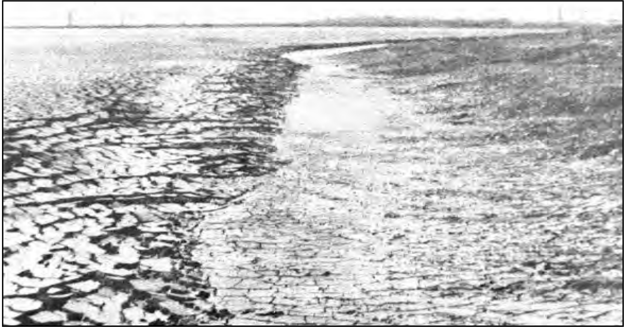
Figure 4-31. Shallow Initial Perimeter Trench Constructed by a Dragline Operating from the Perimeter Dike
