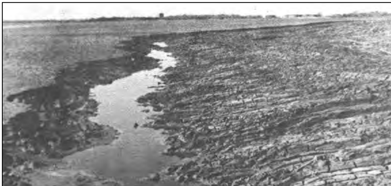
Figure 4-33. Construction of a Ditch 30-45 cm (12 to 18 in.) Deep with Excavated Material Cast on the Interior Slope of a Perimeter Dike
