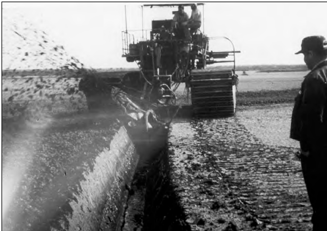
Figure 4-41. Rotary Trenching Device in Operation
